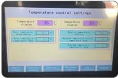
1. PLC control system
